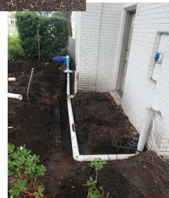
Images are courtesy of River City Gutters and Drainage (904) 330-8658 www.RiverCityGuttersAndDrainage.com
